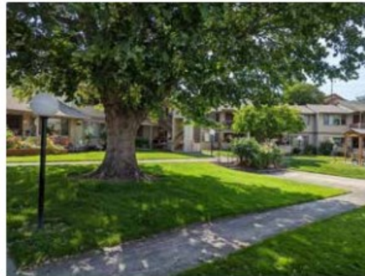
View of subject building exterior and courtyard area.
