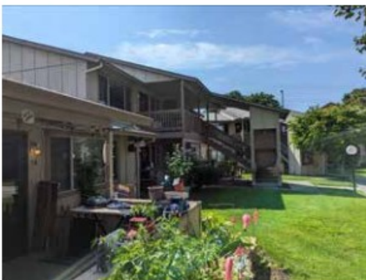
View of subject building exterior.
